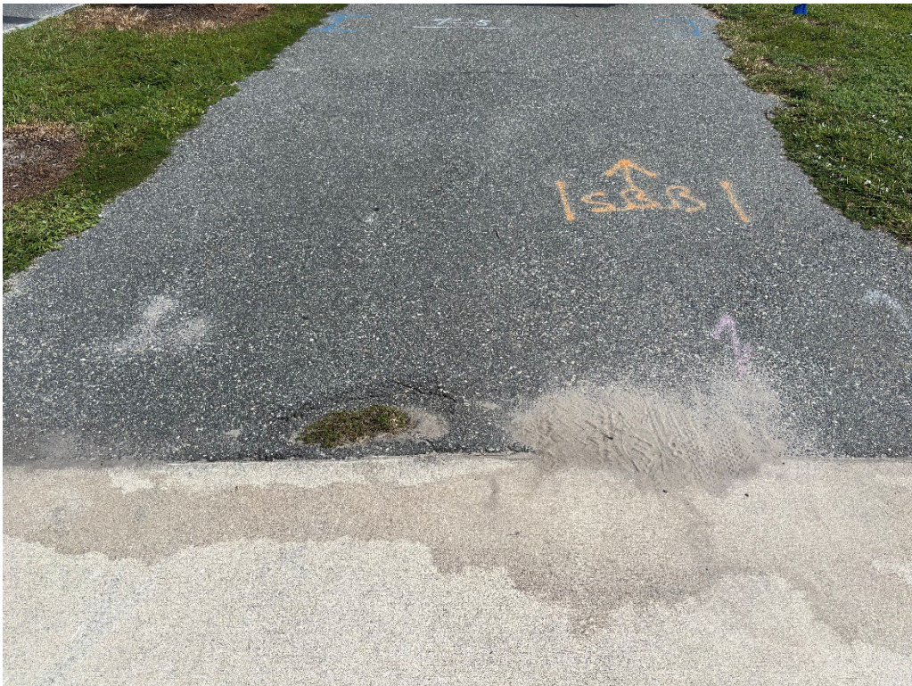
Photo 22 – Asphalt Raveling and Base Failure
