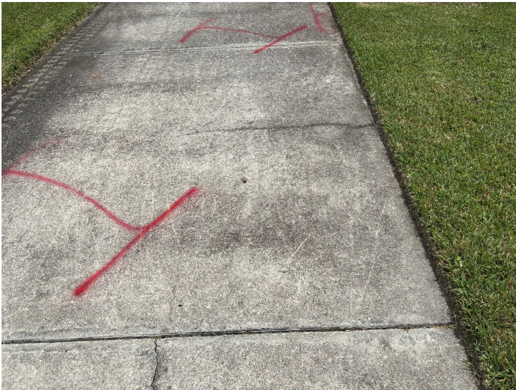
Photo 12 – Surficial Cracked Concrete
