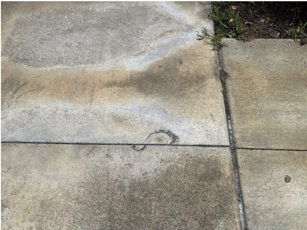
Photo 14 – Surficial Cracked Concrete
