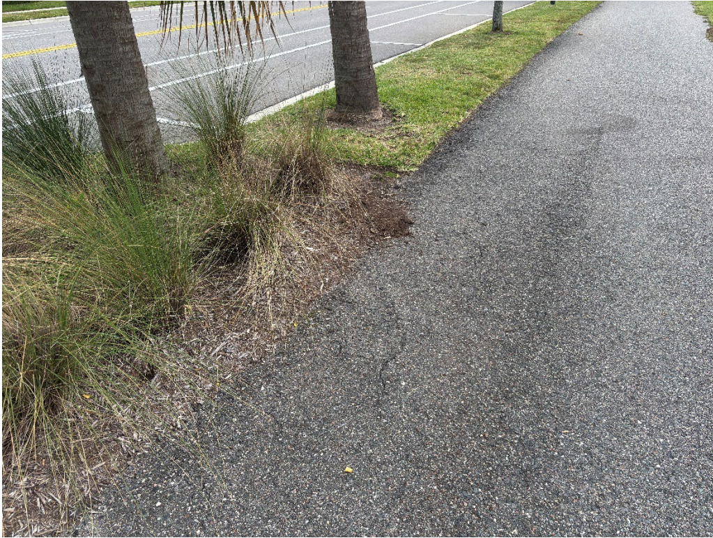
Photo 5 –Asphalt Raveling
