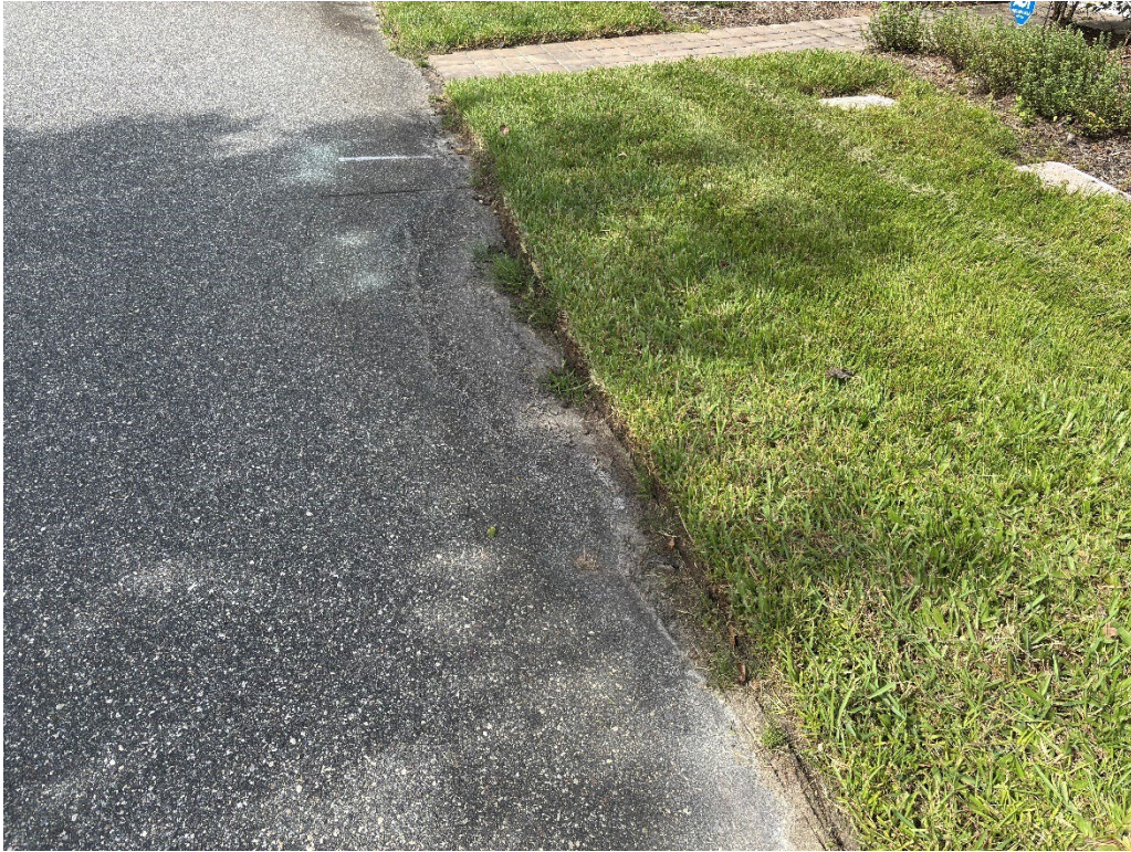
Photo 29 – Asphalt Raveling and Base Failure
