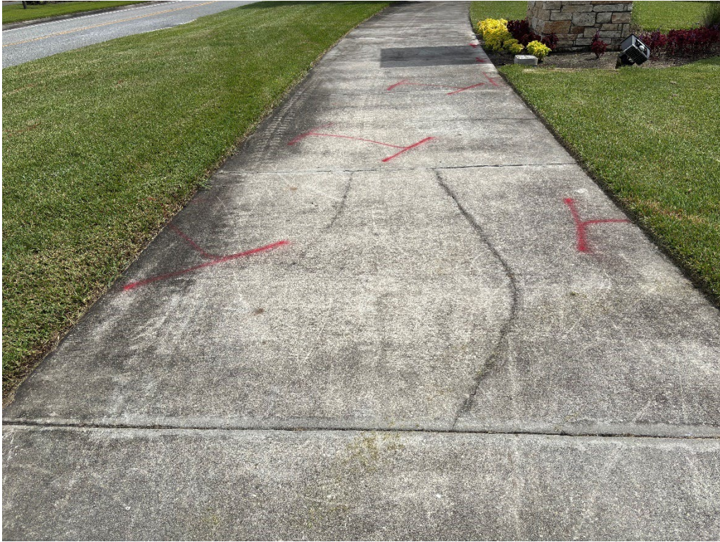
Photo 11 – Surficial Cracked Concrete
