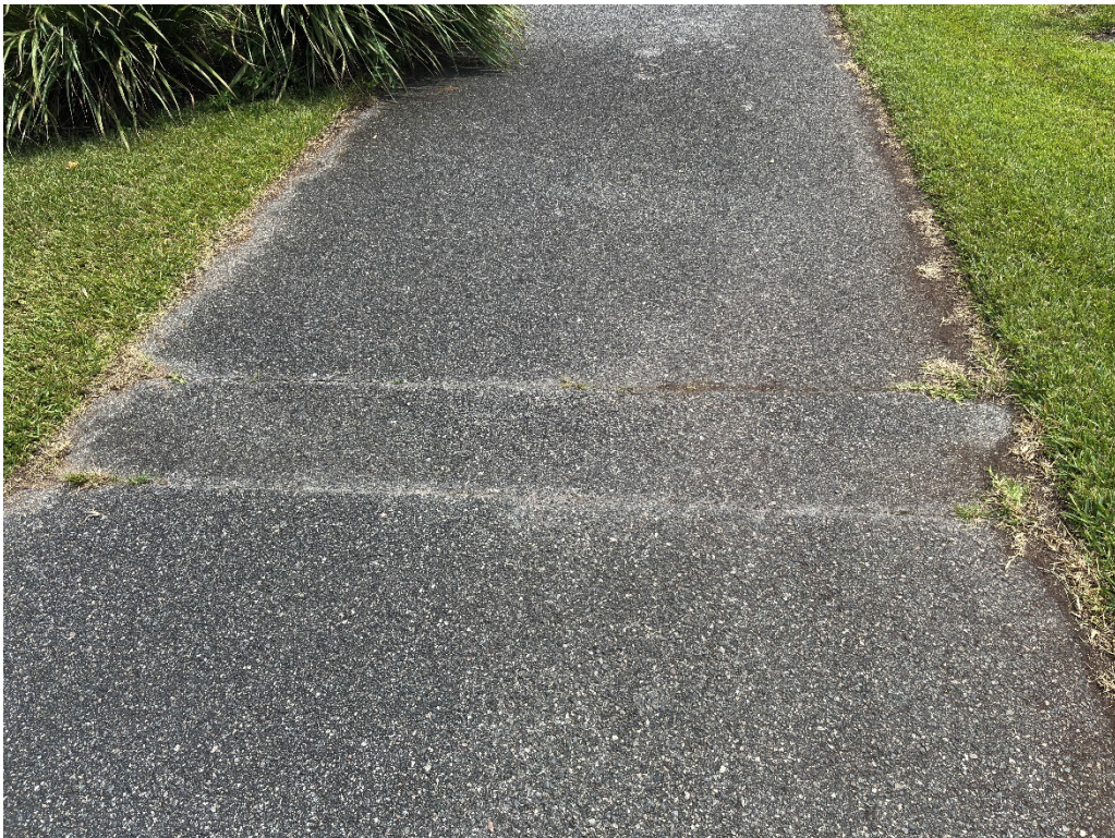
Photo 10 – Poor Quality Asphalt Patch
