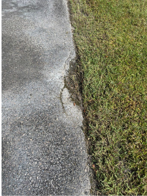
Photo 17 – Asphalt Raveling and Base Failure
