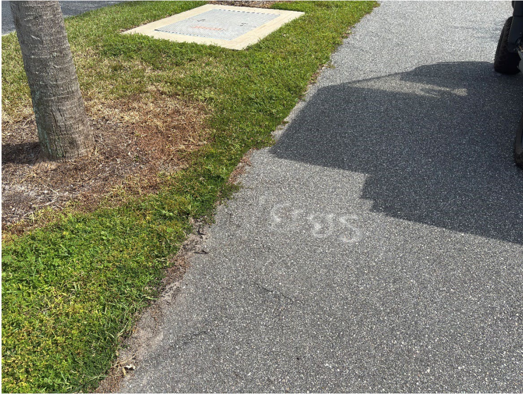
Photo 23 – Asphalt Raveling
