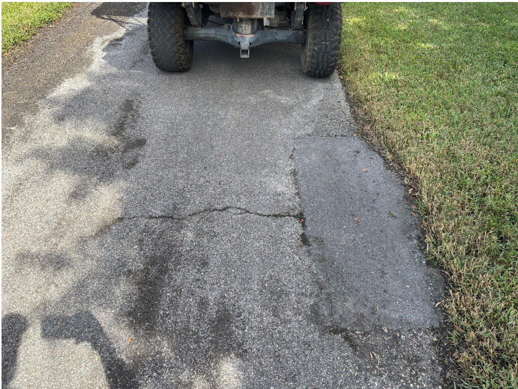
Photo 20 – Poor Quality Asphalt Patch
