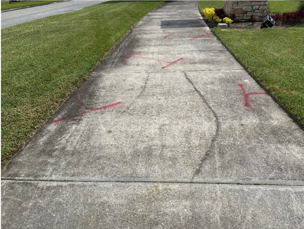
Photo 11 – Surficial Cracked Concrete
