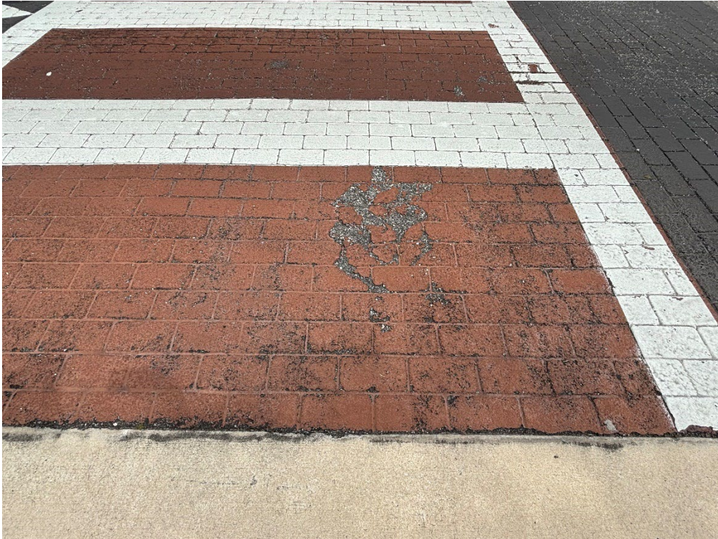
Photo 9 – Deteriorating Thermoplastic and Worn Coloration
