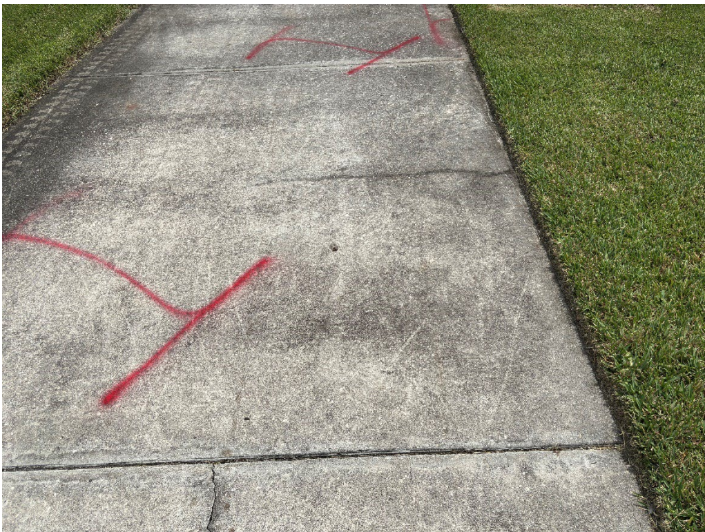
Photo 12 – Surficial Cracked Concrete
