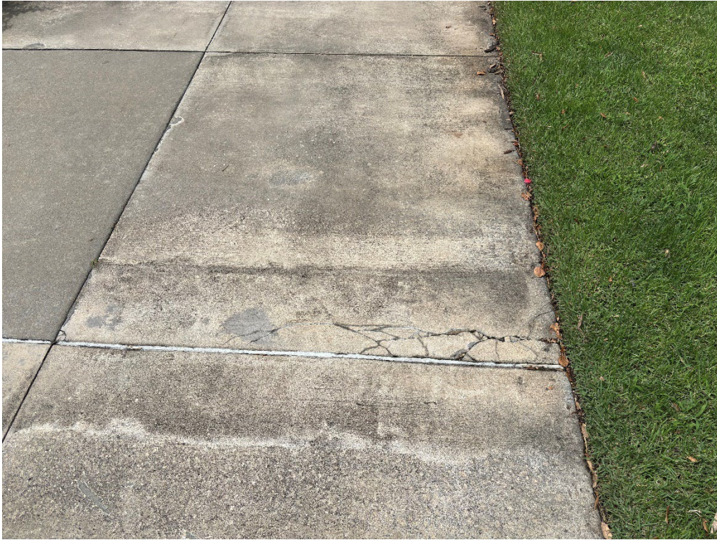
Photo 13 – Surficial Cracked Concrete
