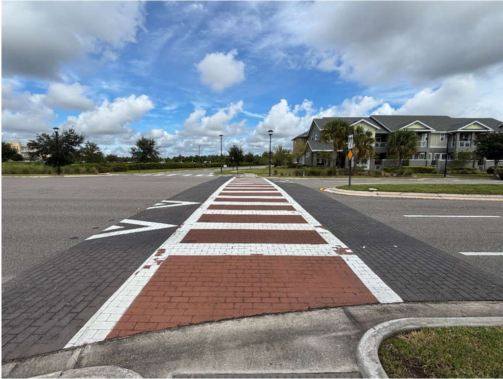
Photo 1 – Deteriorating Thermoplastic
