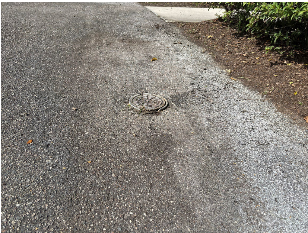
Photo 26 – Valve Cover Reveal 1/2 Inch
