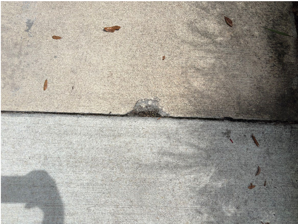
Photo 16 – Broken Concrete
