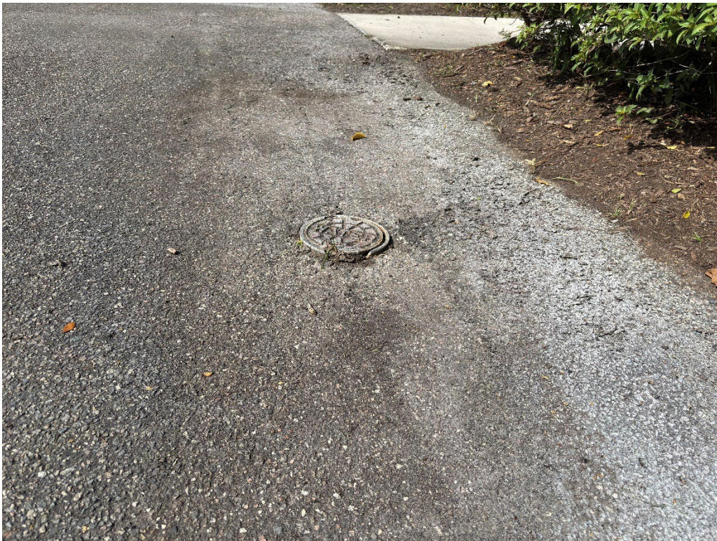
Photo 26 – Valve Cover Reveal 1/2 Inch
