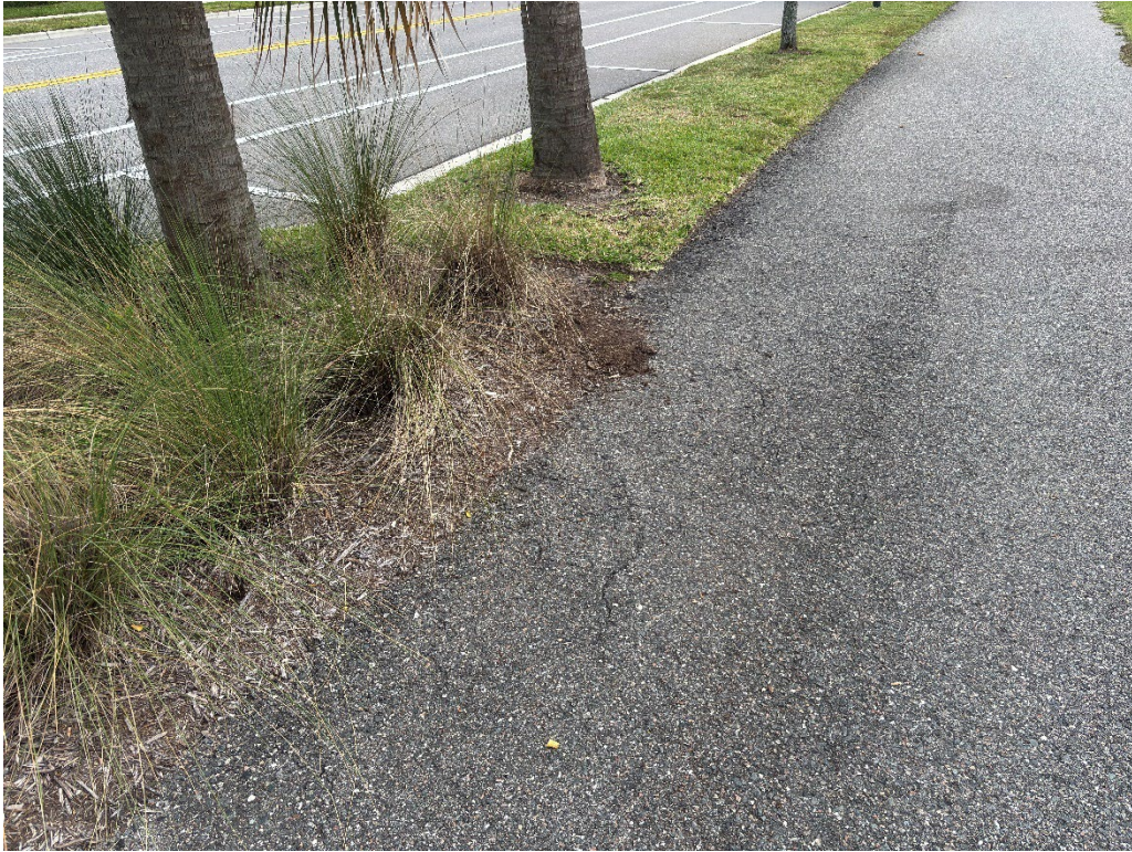
Photo 5 –Asphalt Raveling
