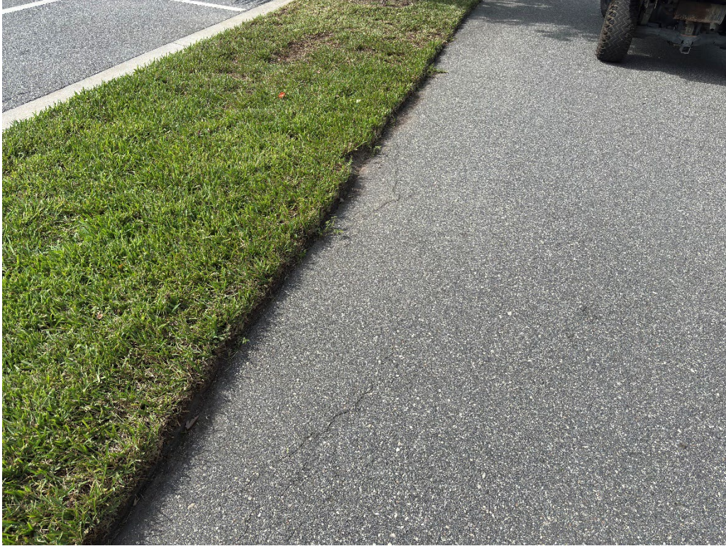
Photo 27 – Asphalt Raveling
