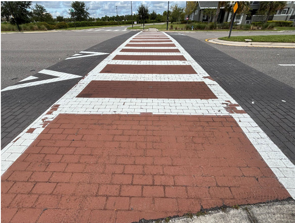
Photo 2 – Deteriorating Thermoplastic
