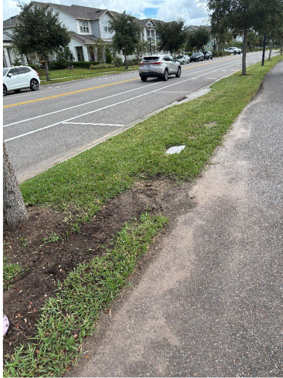
Photo 7 – Low Area Holding Water
