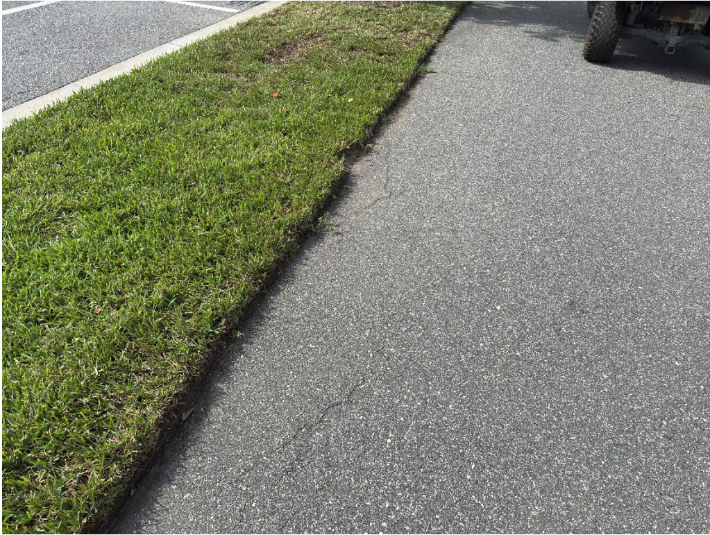
Photo 27 – Asphalt Raveling
