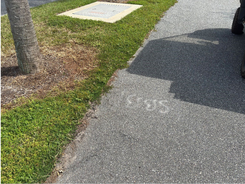
Photo 23 – Asphalt Raveling
