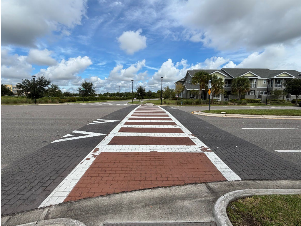
Photo 1 – Deteriorating Thermoplastic
