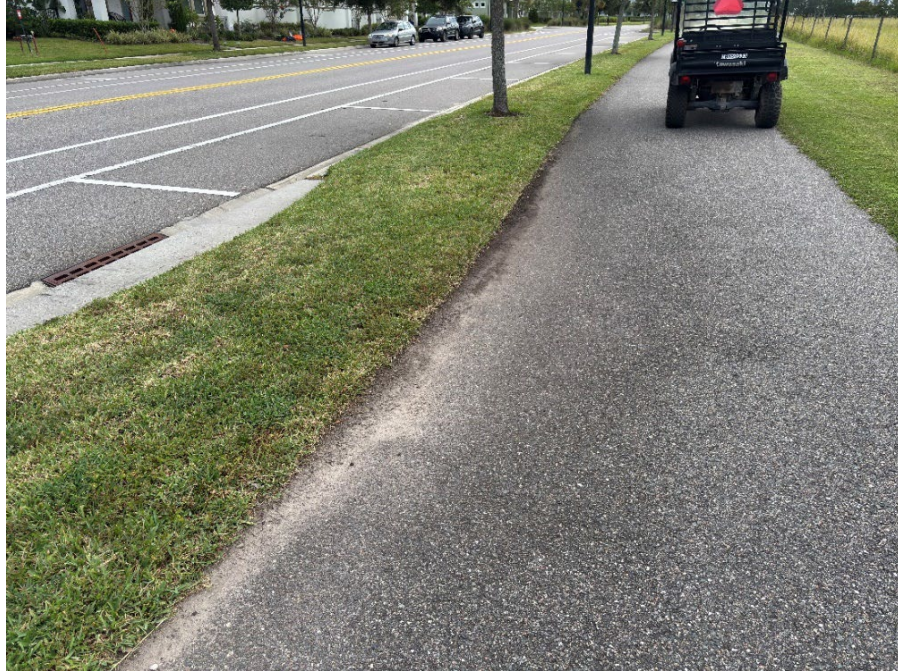
Photo 6 - Low Area Holding Water (No Observed Changes) (Refer to Prior Photo 6 – 2025 Assessment)
