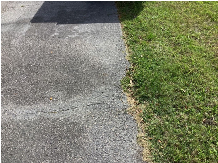
Photo 16 - Asphalt Raveling and Base Failure (Further Edge Failure Observed and Cracked Asphalt from Side to Side) (Refer to Prior Photo 17 – 2025 Assessment)
