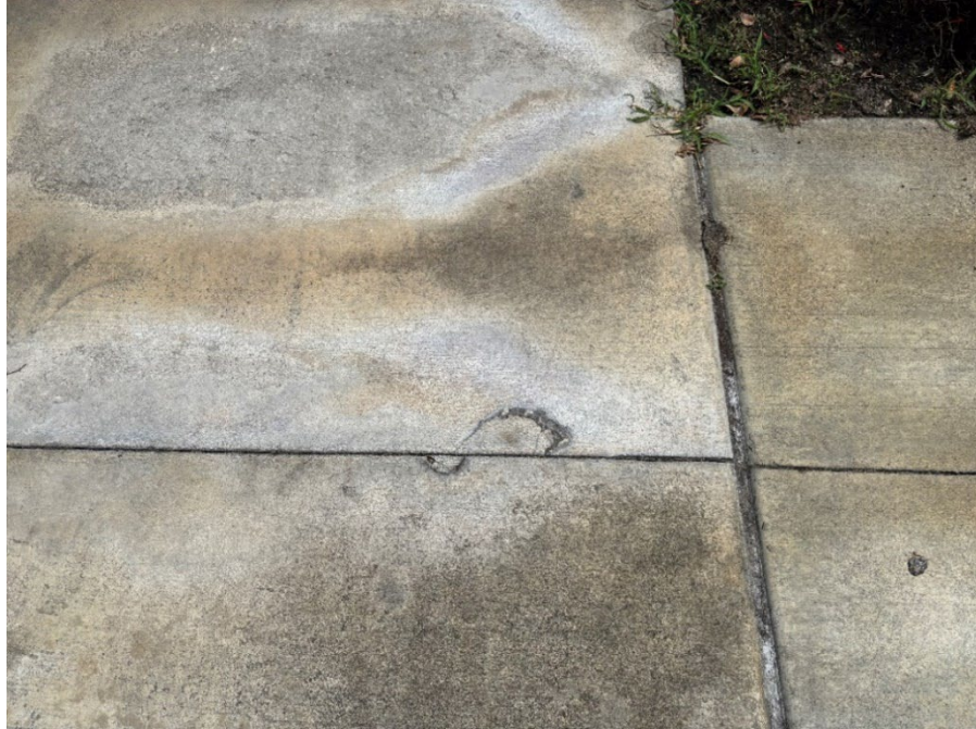
Photo 14 - Surficial Cracked Concrete (No Observed Changes) (Refer to Prior Photo 14 – 2025 Assessment)
