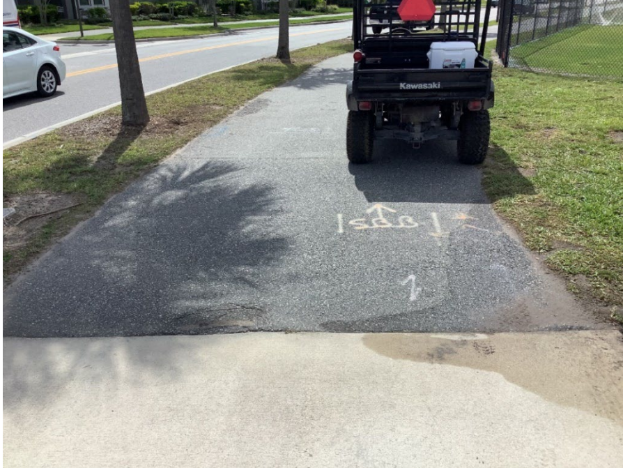
Photo 18 - Asphalt Raveling and Base Failure (No Observed Changes) (Refer to Prior Photo 22 – 2025 Assessment)
