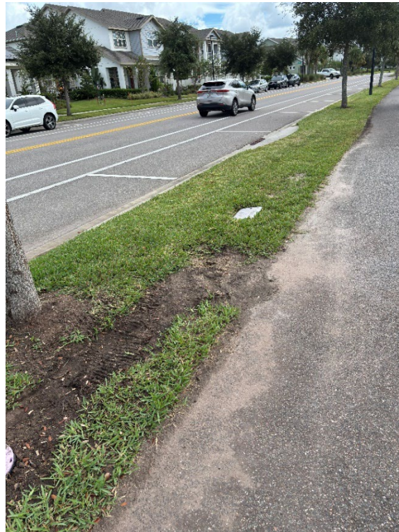
Photo 7 - Low Area Holding Water (No Observed Changes) (Refer to Prior Photo 7 – 2025 Assessment)
