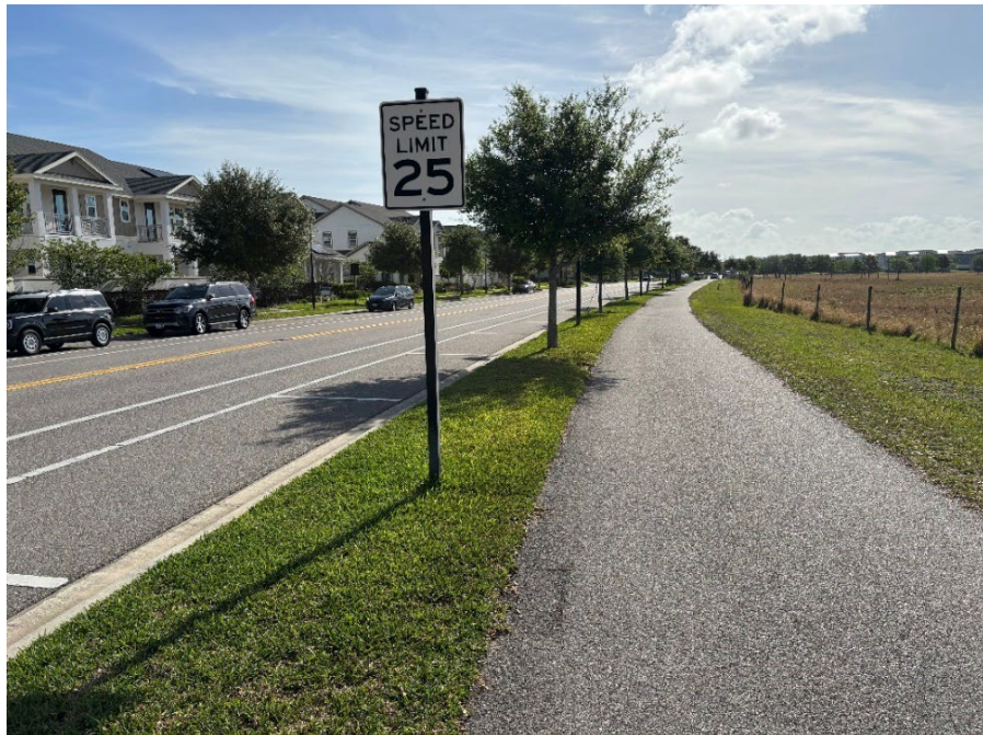
Photo 3.1 – Uneven Asphalt Patch (New Photo – 2026 Assessment)
