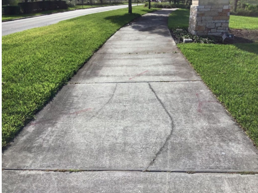
Photo 11 - Surficial Cracked Concrete (No Observed Changes) (Refer to Prior Photo 11 – 2025 Assessment)
