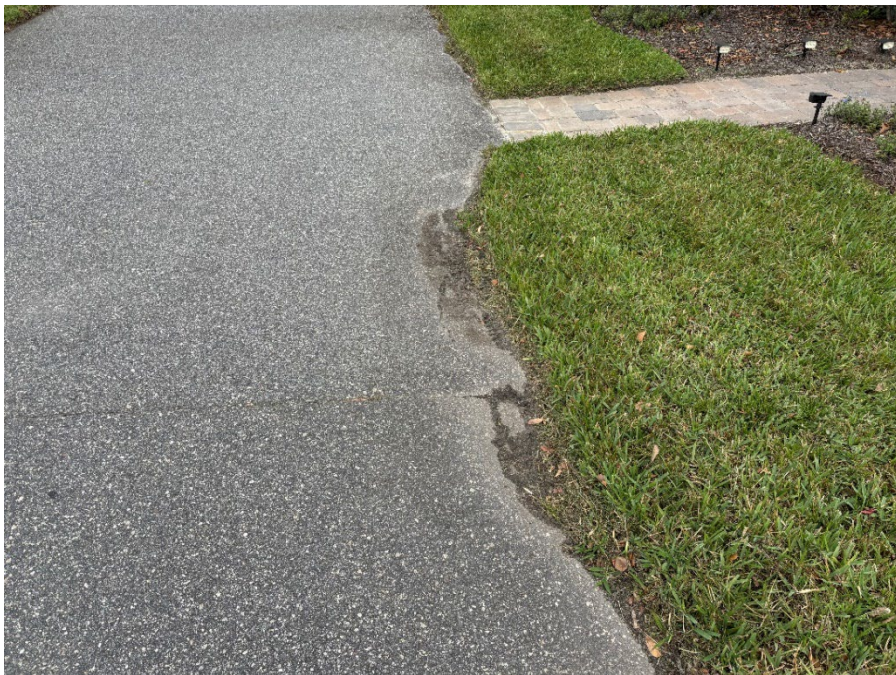
Photo 22 - Asphalt Raveling and Base Failure (No Observed Changes) (Refer to Prior Photo 29 – 2025 Assessment)
