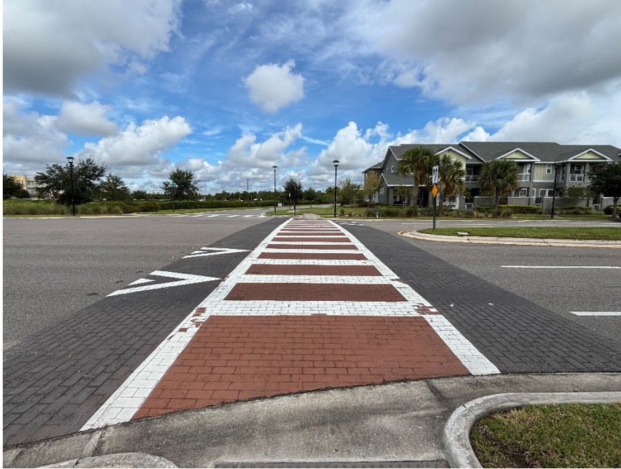
Photo 1 Deteriorating Thermoplastic and Worn Coloration (No Observed Changes) (Refer to Prior Photo 1 – 2025 Assessment)
