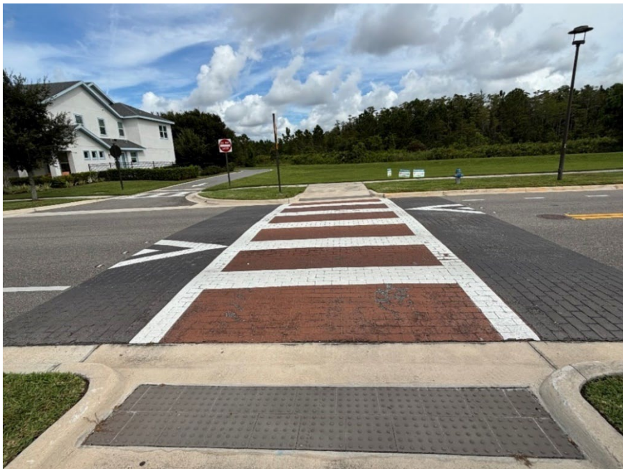
Photo 8 Deteriorating Thermoplastic and Worn Coloration (No Observed Changes) (Refer to Prior Photo 8 – 2025 Assessment)
