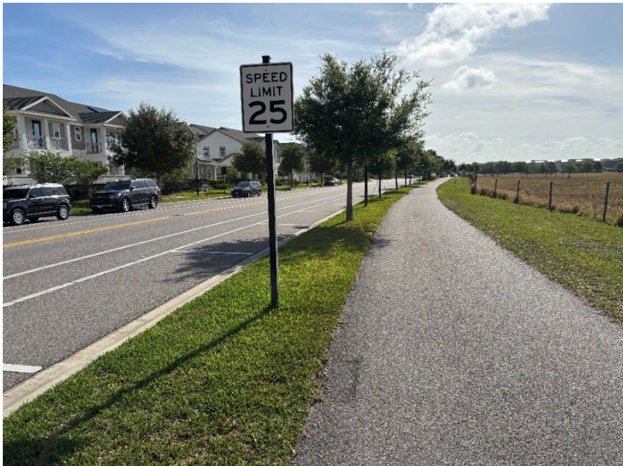
Photo 3.1 – Uneven Asphalt Patch (New Photo – 2026 Assessment)
