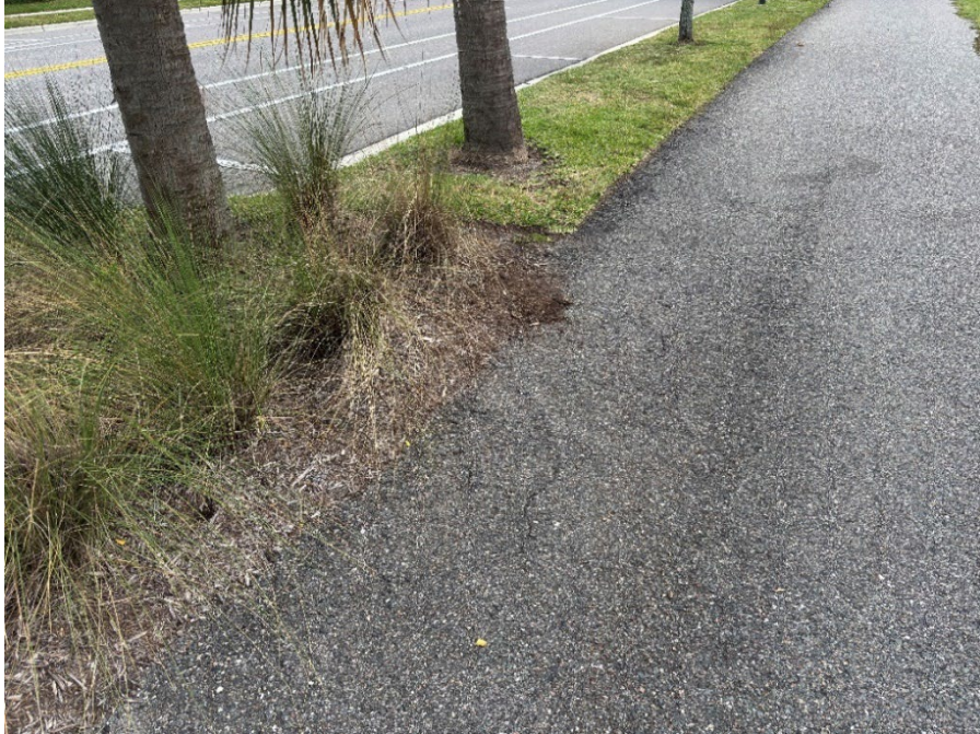
Photo 3 Asphalt Edge Raveling (Increased Asphalt Raveling Observed) (Refer to Prior Photo 3 – 2025 Assessment)
