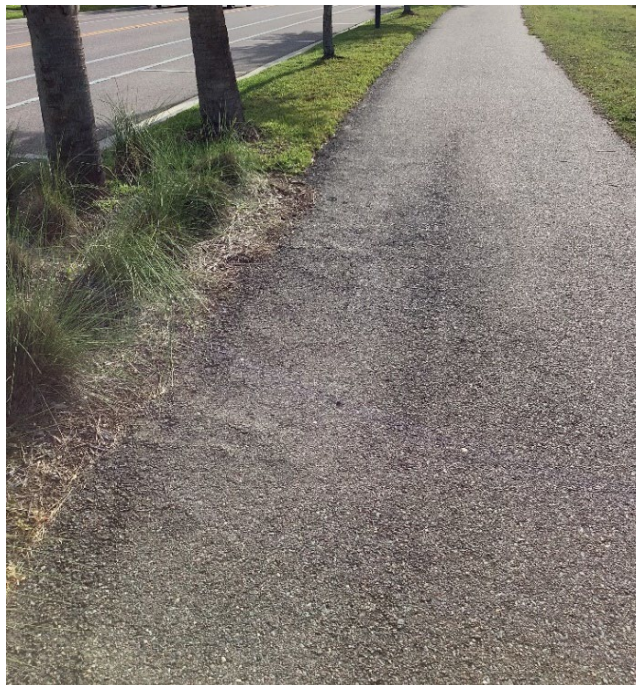
Photo 5 - Asphalt Raveling (Increased Asphalt Raveling Observed) (Refer to Prior Photo 5 – 2025 Assessment)
